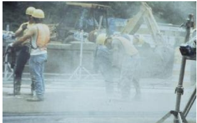
Using multiple jackhammers without dust controls increases silica exposures for both operators and adjacent employees. (Photo courtesy of Kenneth Linch.)
