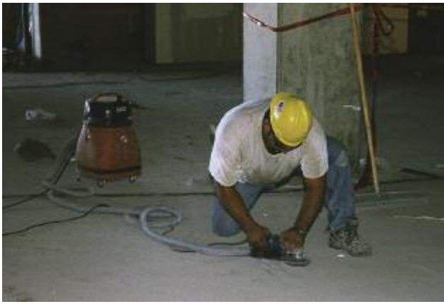
Grinder with attached VDC system. (Photo courtesy of the University of Washington.)
