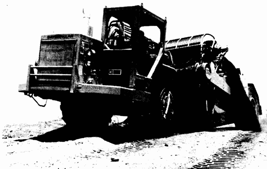
Figure 1-6. Prime Mover Pulling Scraper
