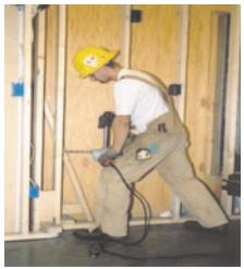
← **SELECT THE RIGHT TOOL.** Choose tools that fit your hand comfortably and have soft grips. A good handle grip prevents your hand from slipping while using the tool. Consider using tools that reduce the amount of force or movements you use. Keep tools well maintained.
